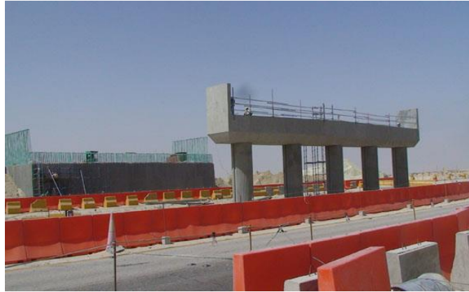
Figure 9: Manifa Bridge (Aramco, 2017).
