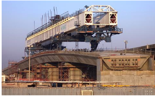
Figure 7: Precast Dammam Bridge (Freysinet, 2022a).
