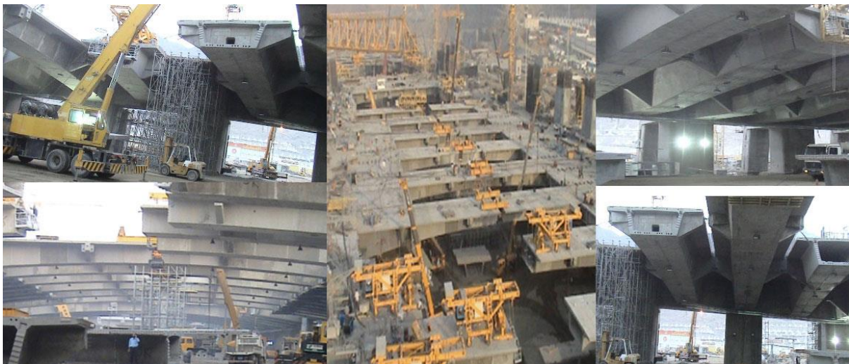
Figure 11: Improvement of Al-Jamarat Bridge (Freysinet, 2022b).
